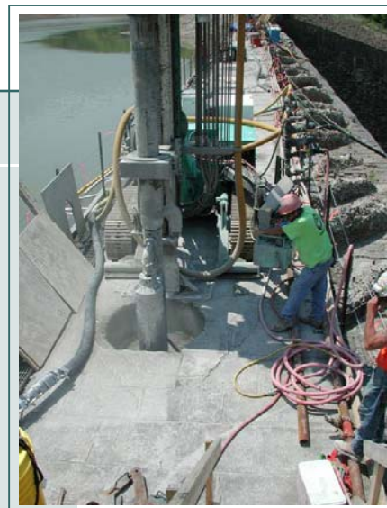
Installing post-tension anchors at Gilboa Dam
