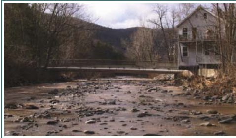
Reach beneath Rt. 214 bridge in Phoenicia
