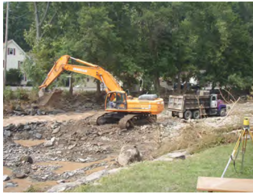
Above: An excavator removing excess gravel from the Stony Clove in the days following the flood.
