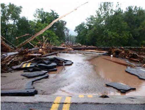
Left: Bridge Street Bridge in Phoenicia shortly after Hurricane Irene flood waters began to recede. Notice how much the double yellow line moved because of the force of the flood waters
