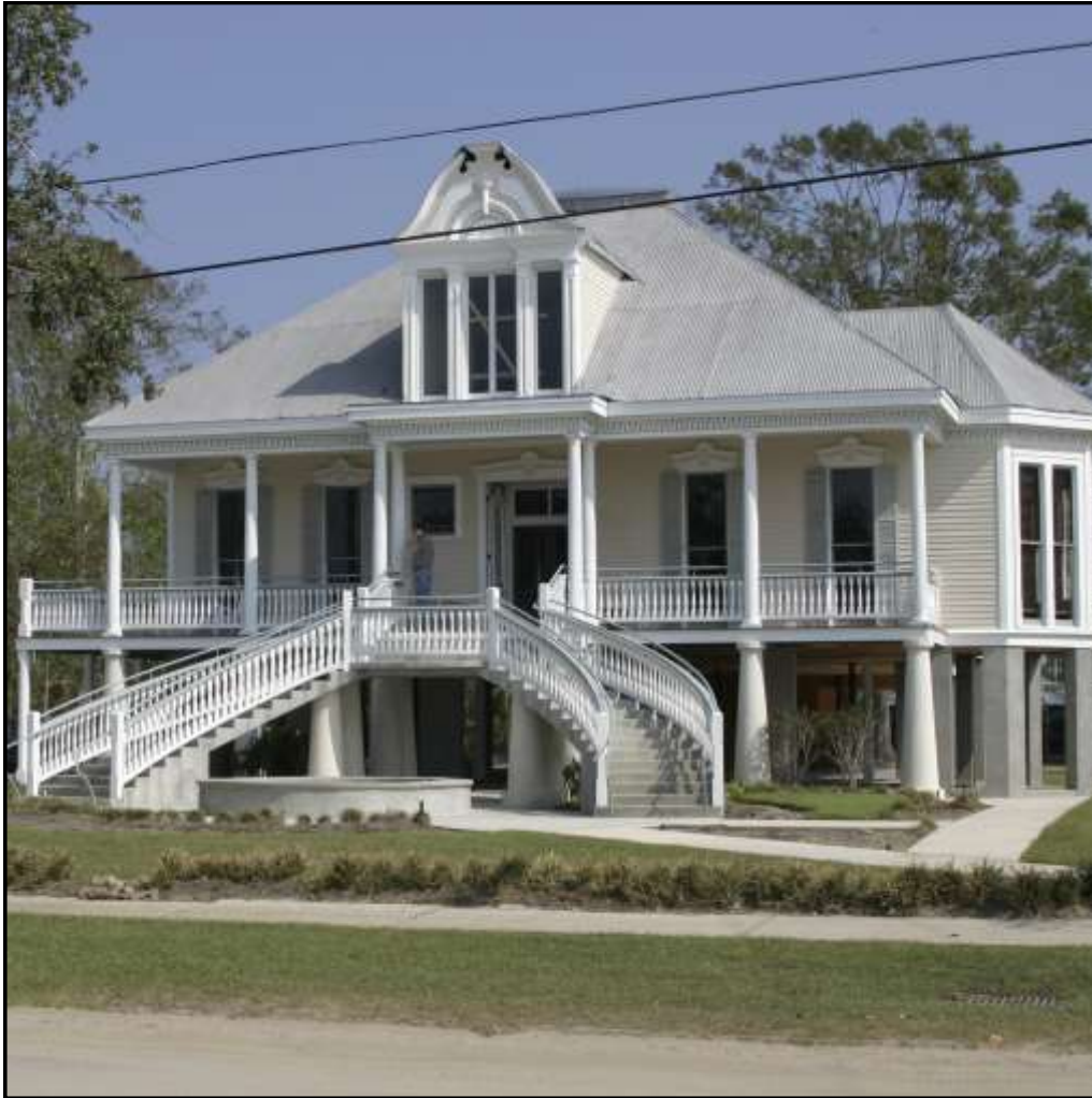
Above: An example of a home built on columns. Elevated homes are significantly less susceptible to flood damage and cost less in flood insurance premiums.
