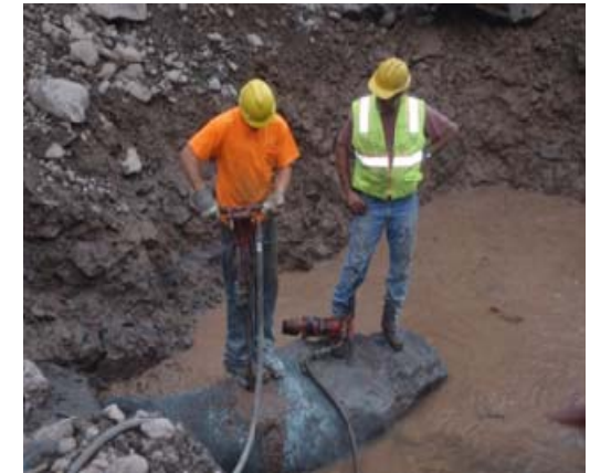
Rocks pinned to bedrock with steel rebar
