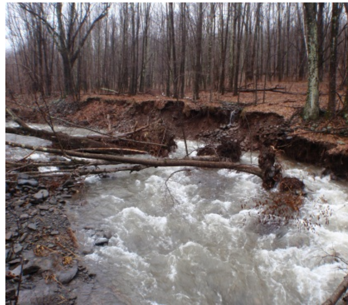
Bank erosion from trees that were not cut before falling into the stream
