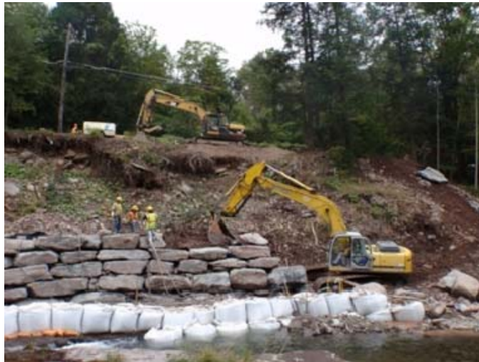
Rock is placed at the toe of the eroding slope on Woodland Creek. Large sand bags prevent construction runoff into the stream
