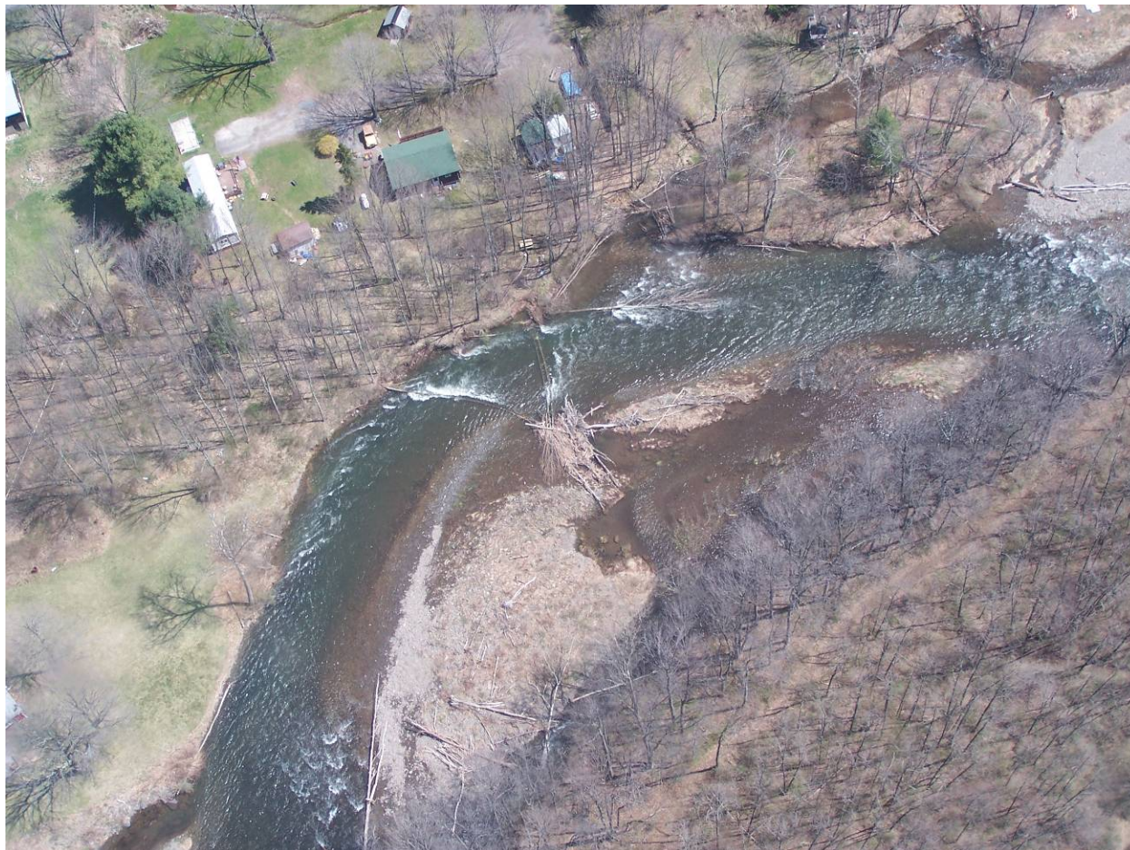
Esopus Creek (Reach 9) depicting several stream management concerns, Ulster County, NY (April, 2009)
