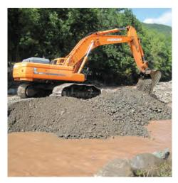
Removal of a mid-channel gravel bar as part of planned channel restoration on the Stony Clove Creek in Phoenicia, NY, September, 2011.
