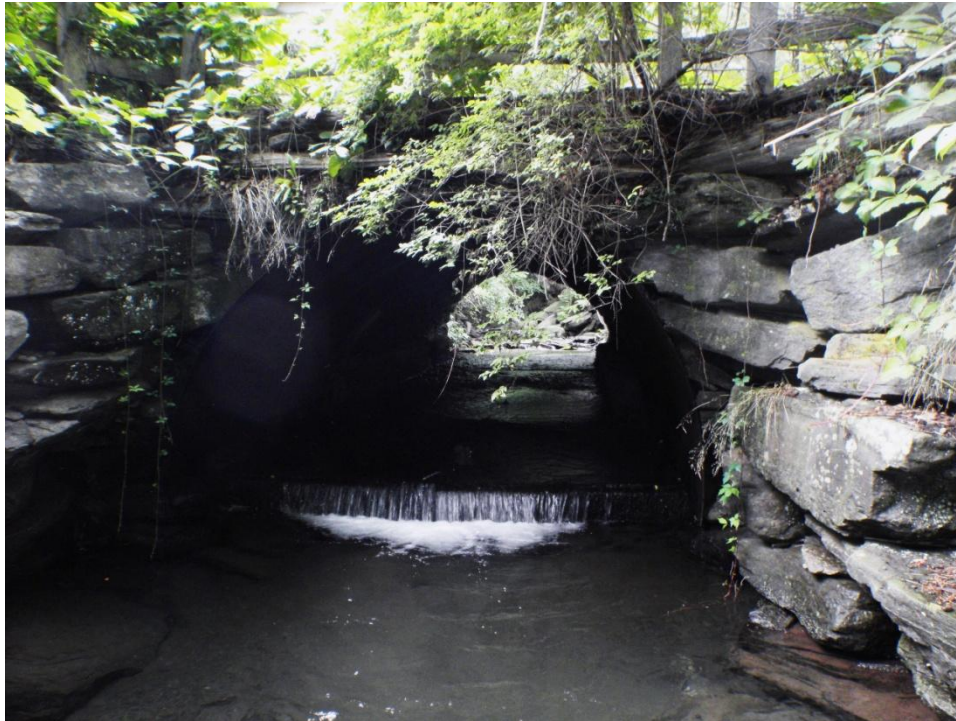
Figure 11: The observable section of stream has been straightened and constricted, conveying flow through a culvert and stacked rock walls to protect roadway infrastructure.
