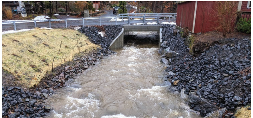
An upsized culvert on DeSilva Road constructed by the Town of Olive in late 2020 performed well during the Christmas Day flood. Photo by Ethan Ely
