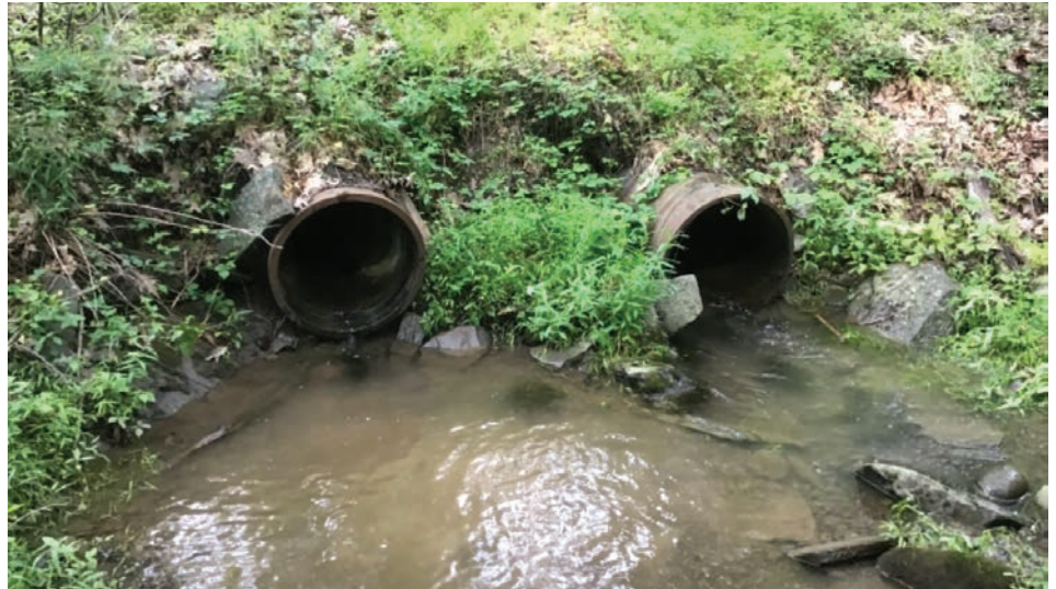
A scour pool beneath two under-sized culverts with evidence of erosion.
