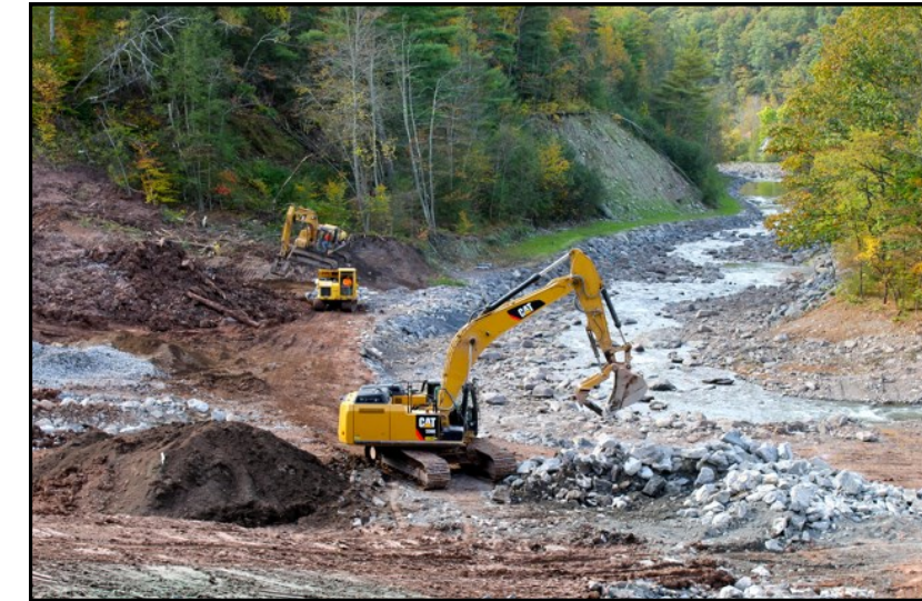
Above: Rocks are placed along the toe of a large hillside along the Stony Clove Creek in Chichester. The project treated one of the largest sources of suspended sediment in the Upper Esopus Creek system.
