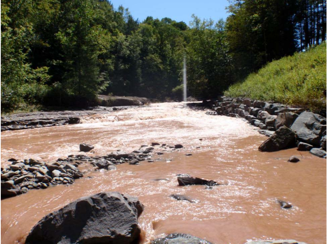
Figure 6 Post-Hurricane Irene (9/4/2011). Observations indicate rock wall and bio-engineered slope no damage.
