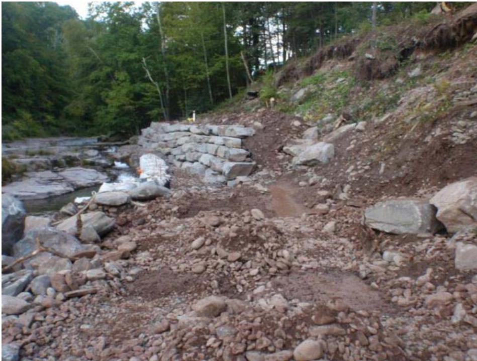
Figure 7 Construction of pinned and stacked rock wall to stabilize hillslope failure.
