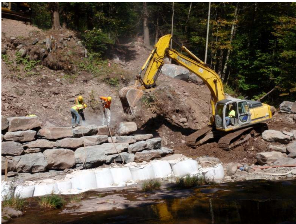
Figure 10 Construction crew using jack-hammers to pin stone wall together with rebar.
