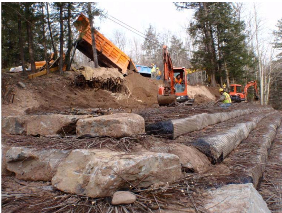
Figure 14 Construction of the bio-engineering soil slope, VRSS 2
