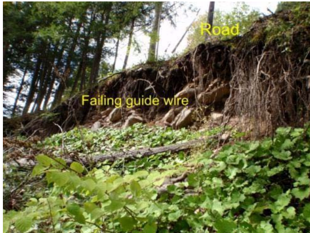
Figure 1 Eroding stream bank and area of undercut road.
