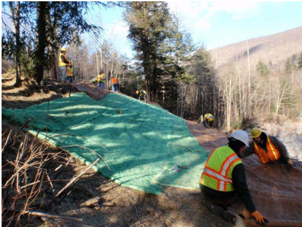
Figure 16 Application of erosion control matting
