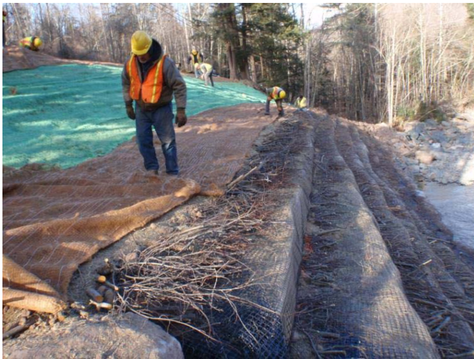
Figure 17 Erosion control matting 2
