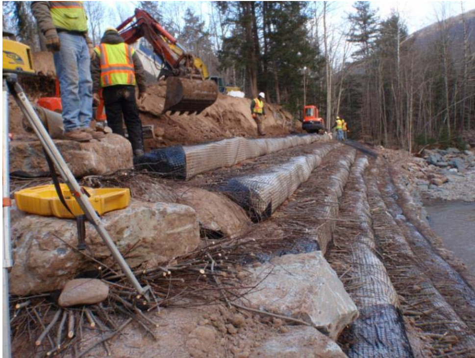
Figure 13 Construction of bio-engineering vegetated reinforced soil slope (VRSS). Nov 2010
