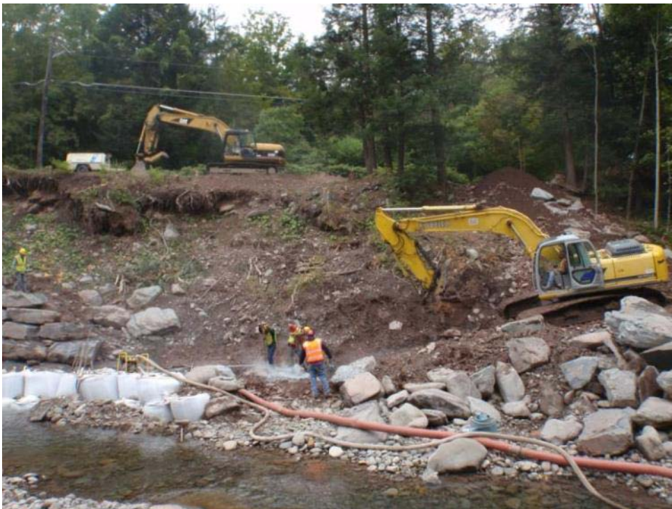
Figure 8 Setting the stacked rock wall deep, keyed into stream bed.
