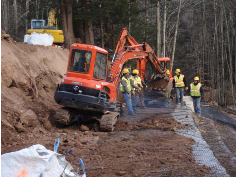
Figure 15 Construction of VRSS 3
