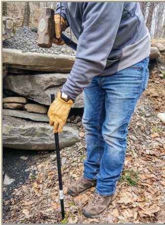
Use form pin to create a pilot hole.
