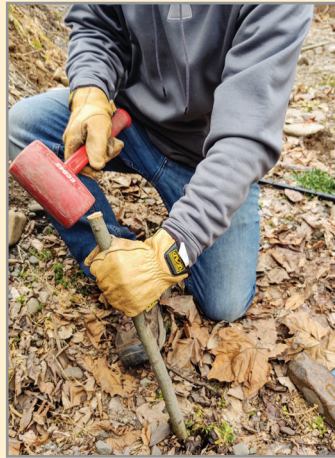
Drive stake into soil using a dead blow hammer or mallet.
