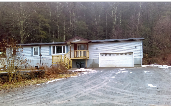
A home near Phoenicia, NY elevated on extended foundation walls. Photo: AWSMP
