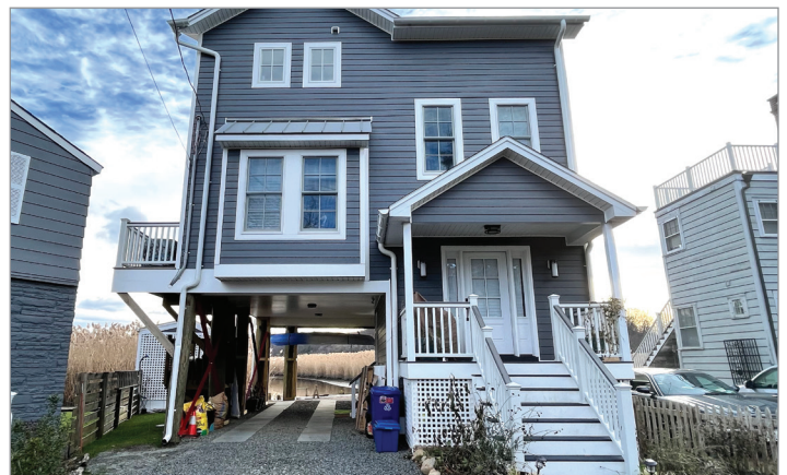
A home elevated on piers; reconstructed after Hurricane Sandy to meet current NFIP standards. Piermont, NY. Photo: AWSMP
