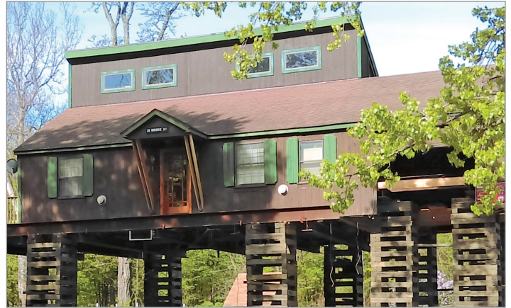
A home in Phoenicia, NY undergoing an elevation. Photo: AWSMP
