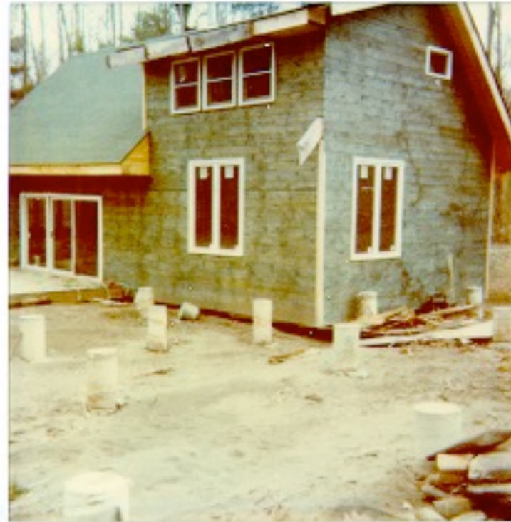
01-04-24-96 (T) CHARLESTON END OF BUTLER DR - ADJACENT
