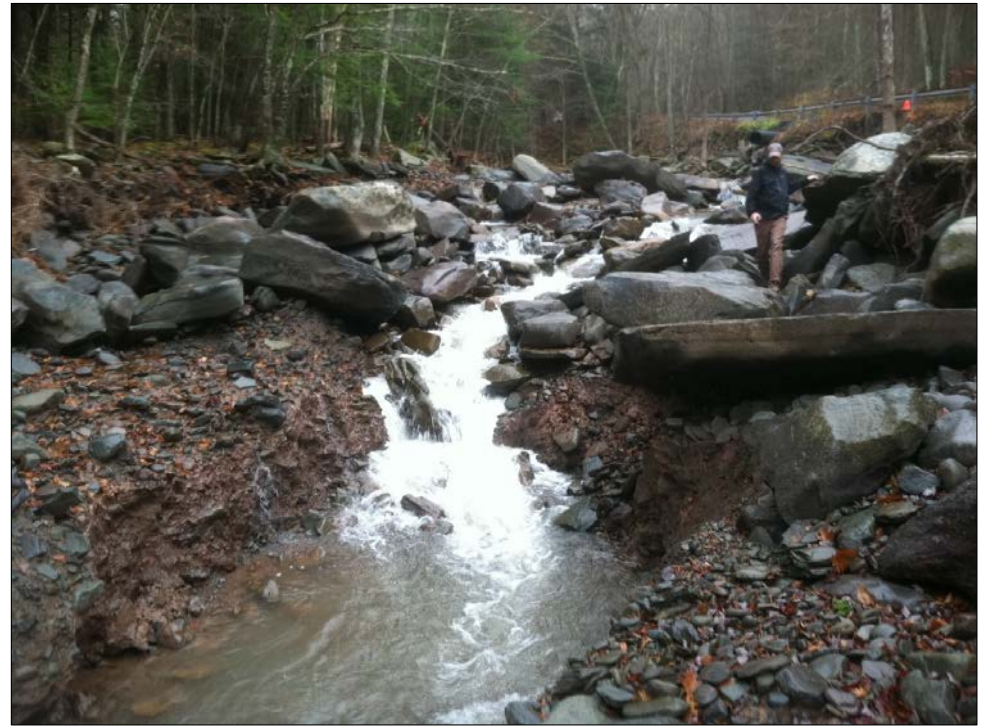
TS Irene Flood headcut, Warner Creek, Esopus Creek Watershed
