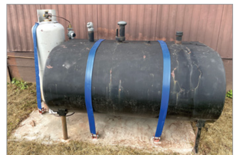
An anchored fuel tank near Halcottsville, NY. Photo: CWC.
