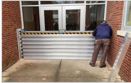
A staff member at Townsend Elementary School in Walton, NY practices installation of a removable flood barrier at one of the building entrances. Photo: CWC.
