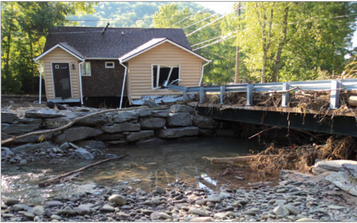
A flooded home pushed off its foundation by floodwaters, Oliverea, NY. This home was not elevated or wet floodproofed. Photo: A Bennett
