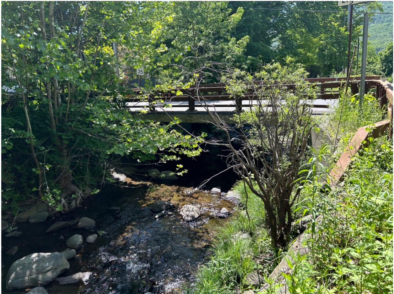
Eighmey Road crossing.
