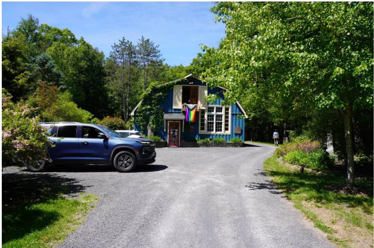
Cox Gallery located in floodway. Beaver Kill located off picture right.
