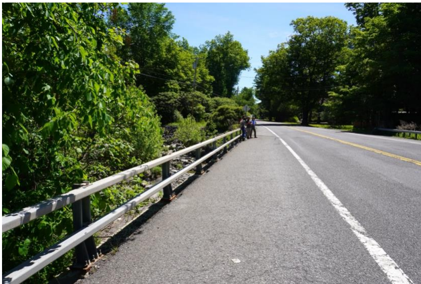
NY-212 crossing over Beaver Kill near Lake Hill (fifth bridge) at sharp valley slope break with resulting deposition.
