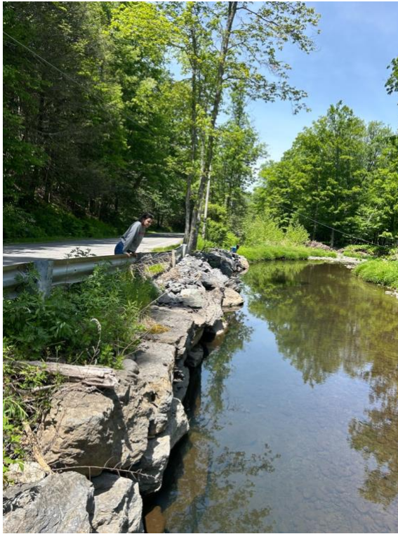
Rock wall along Sickler Road where road and stream interact.
