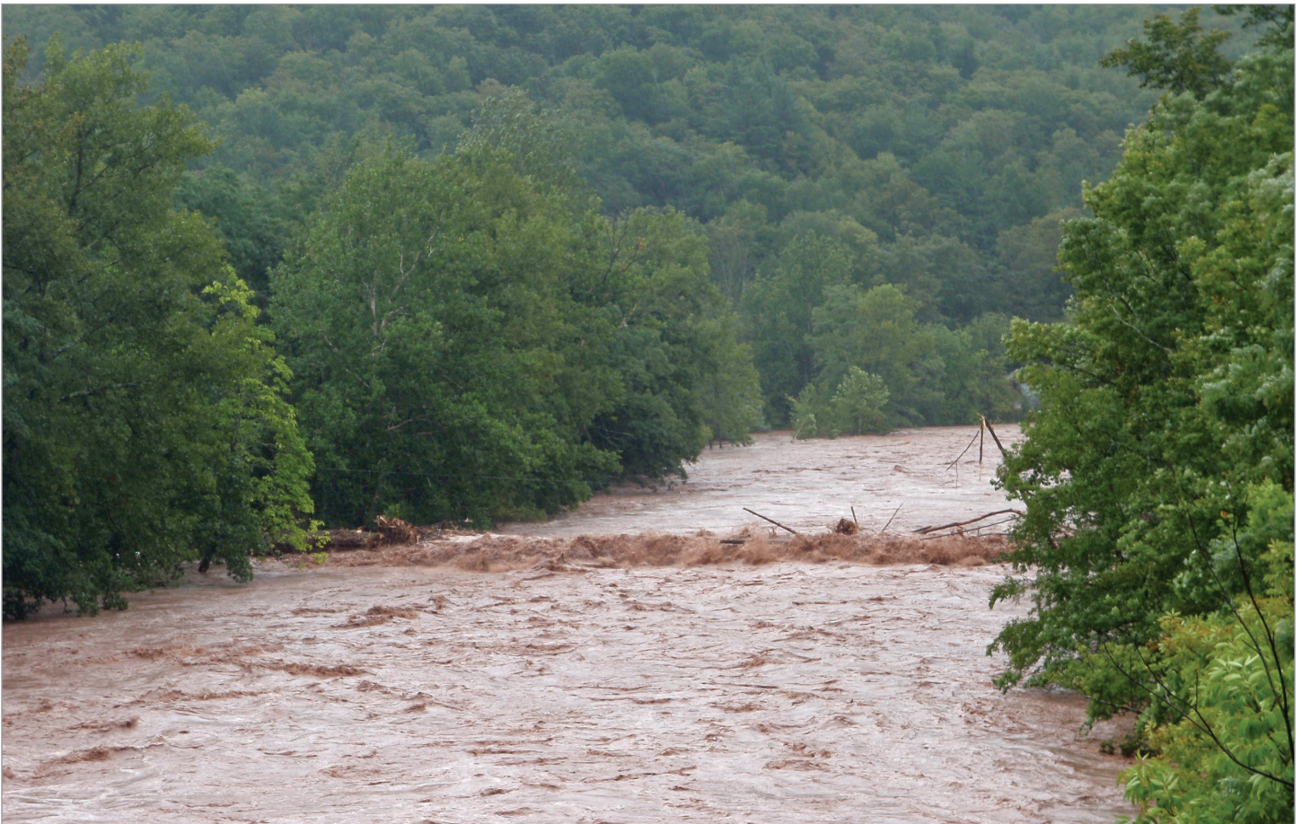
The Bridge Street Bridge in Phoenicia being overtopped by floodwaters as a result of Tropical Storm Irene (2011).
