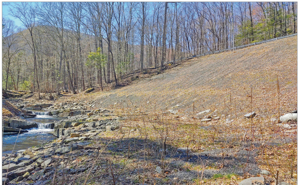
A floodplain was created on this section of the Bushkill and planted with woody vegetation to prevent erosion into Watson Hollow Road.
