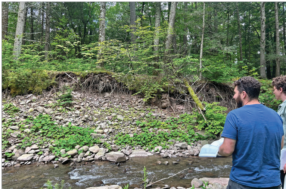
AWSMP staff review stream restoration plans facing an eroding hillslope on Broadstreet Hollow. The stream site near Allaben, NY will be restored to stable and healthy conditions this summer.
